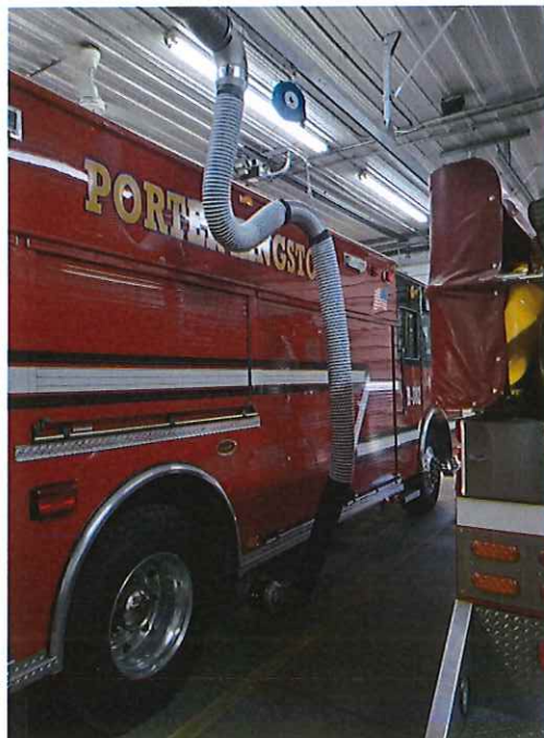
Exhaust Coupling Attached To Vehicle
